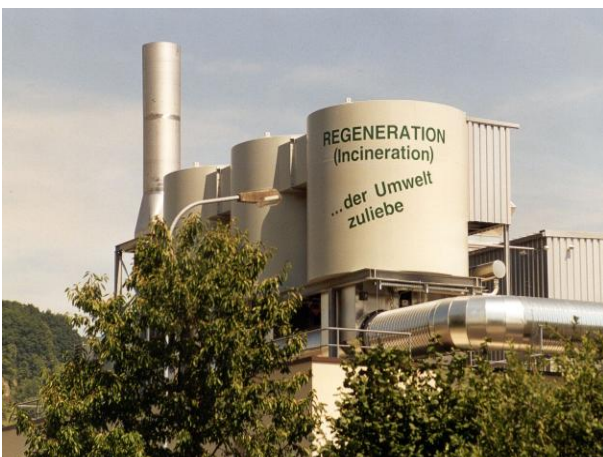
Incinerator in Europe
